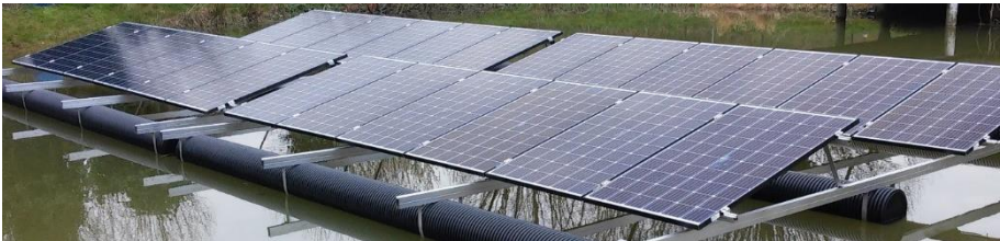
Fig. 3. Pontoon system by Ministry of Solar [3]
