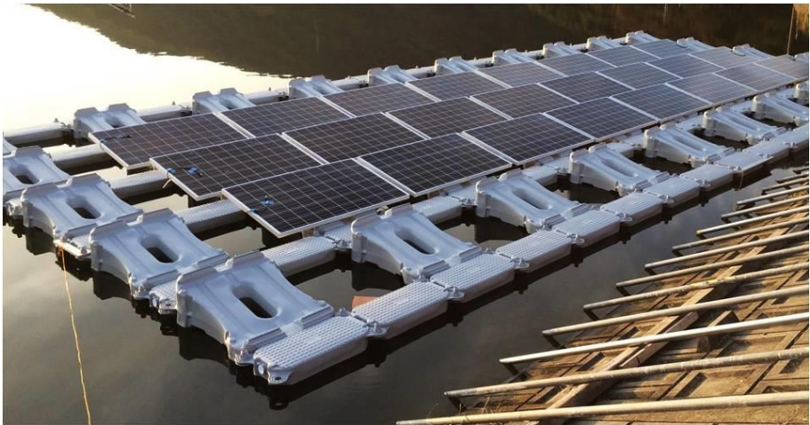
Fig. 2. Pontoon Hydrelío® system by Ciel&Terre [29]
